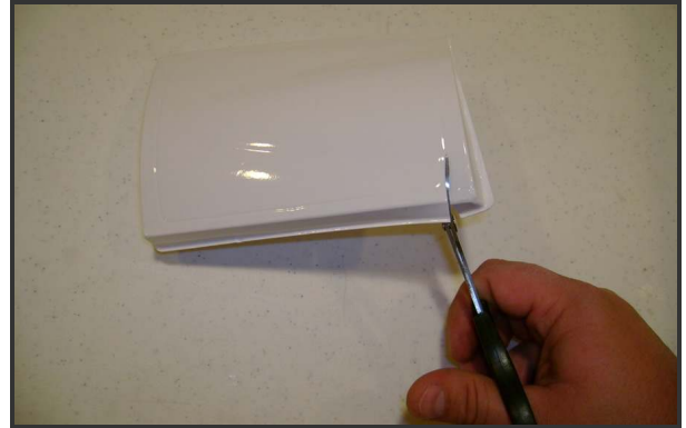
Trim the fan access hatch cover
